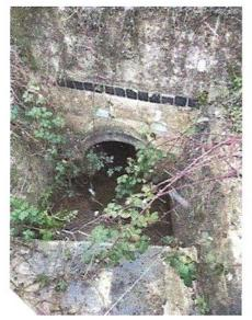
Silt, rubbish & overgrowth is still evident within the outlet and the Reen proceeding this outlet... (see previous two photos and left)
