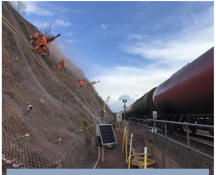
Work is ongoing to stabilise the cutting at Little Haglow
